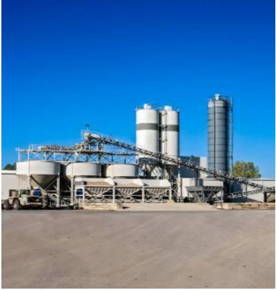
Cement manufacturer Optimize clinker-kiln operations with AI at Edge
