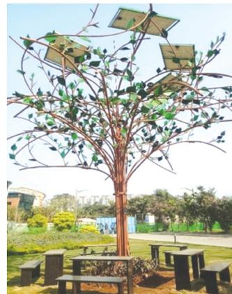
Taking inspiration from the natural environment, India's Corporate Real Estate Services team also created and installed the first ever solar tree (pictured left) at our Airoli campus in Mumbai. The unique tree-like structure has a functional power generator that mimics a tree trunk with solar panels acting as leaves.
